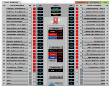
web-based power metering interface (PMI)
